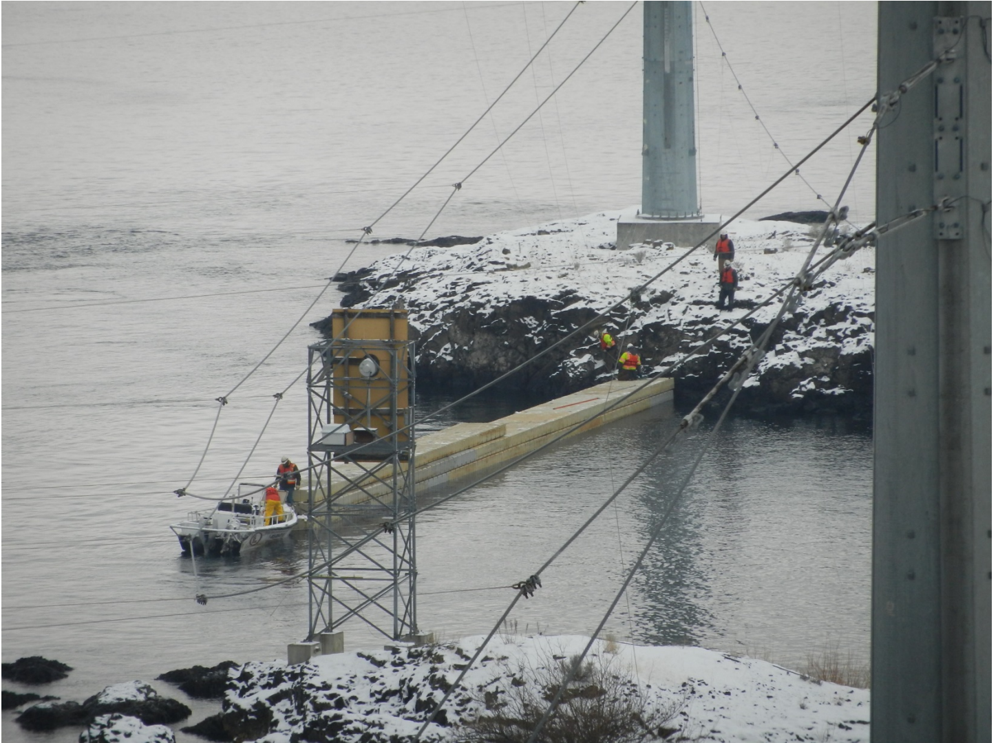
Installing a Temporary Dock for 2018 Avian Lines Replacement (December 2017)
